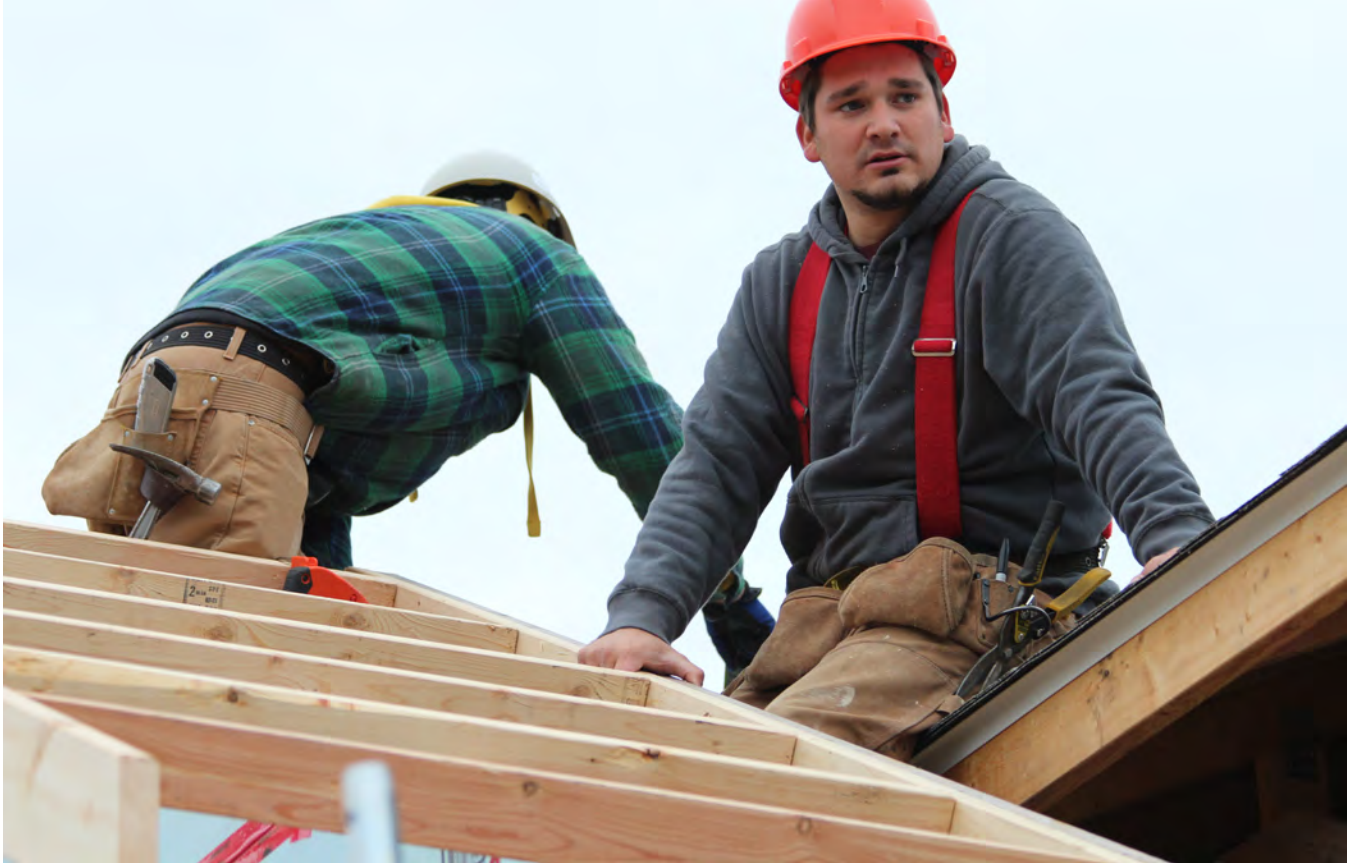
CONSTRUCTION STUDENTS WORK ON BUILDING A NEW RESIDENTIAL HOUSE
