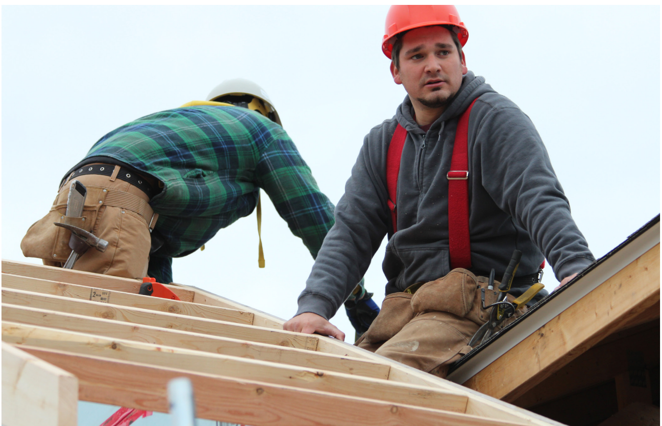
HOME INSPECTION STUDENTS INSTALL THE ROOF ON A RESIDENTIAL HOUSE LOCATED ON THIRD LINE IN SAULT STE. MARIE
